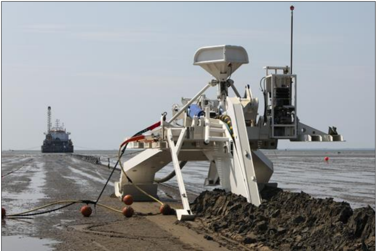
Figure 6-1: Example of Cable Plough Installing Shore End Cable
